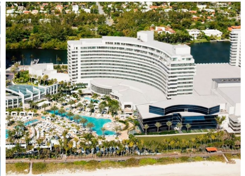
Sorrento Tower at Fontainebleau, Miami Beach, FL
